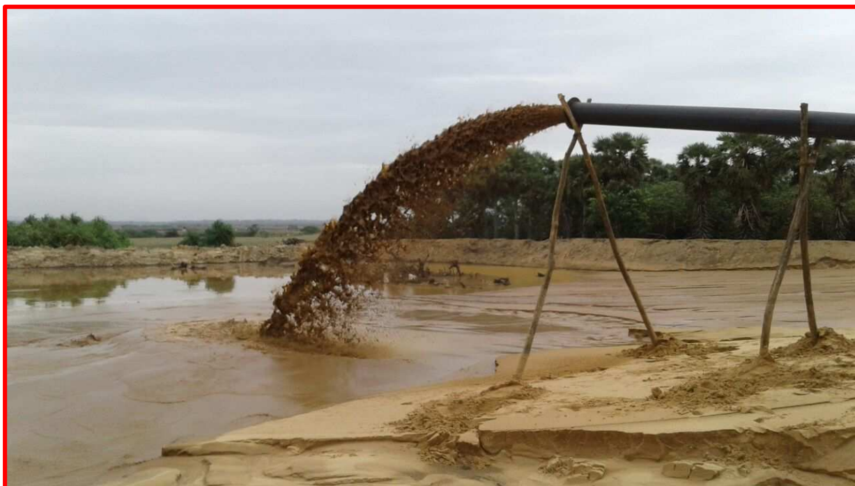
BACKFILLING OF MINED OUT AREA
